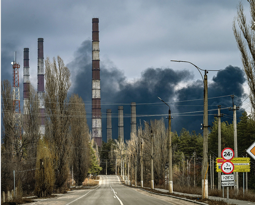
Smoke rises from a shelled power plant outside the town of Shchastya, near the Ukrainian city of Luhansk, on 22 February 2022.
