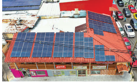
←↑↔↘↙ Rooftop solar power totaling about 200 kilowatts, complemented by 1 megawatt-hour of battery storage, supplies electricity to 14 businesses in Adjuntas.
