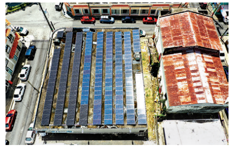
←↑↔↘↙ Rooftop solar power totaling about 200 kilowatts, complemented by 1 megawatt-hour of battery storage, supplies electricity to 14 businesses in Adjuntas.
