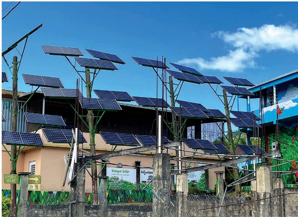
→ The Solar Forest, a novel installation of PV panels, doubles as a public charging station in the town square of Adjuntas.
