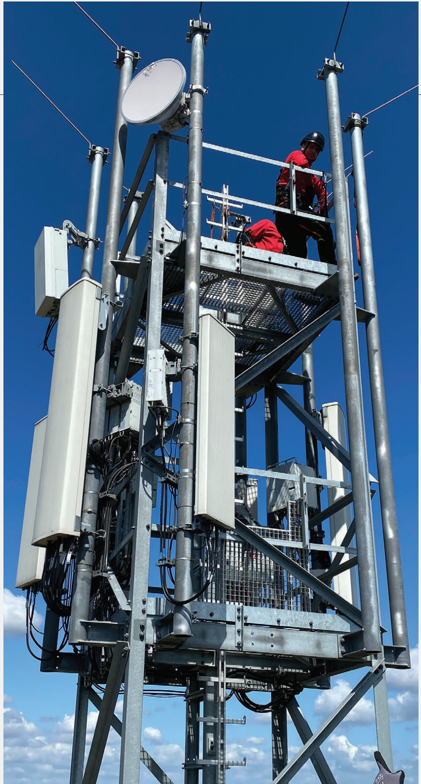
This 5G cellphone tower undergoing installation in Germany in 2020, uses a proprietary system called a radio access network (RAN) that transmits, receives, and processes wireless data. Efforts are now underway to open up RANs to provide greater versatility and access.
