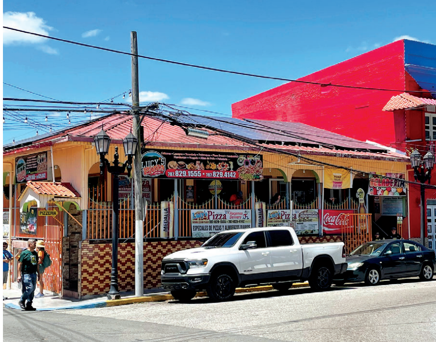
↑ The pizzeria in Adjuntas is connected to a microgrid. It should still be able to operate even if the main power grid goes down.
