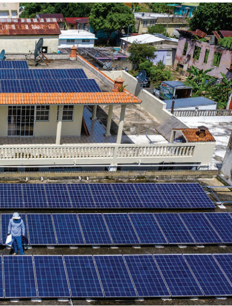
←↑↔↘↙ Rooftop solar power totaling about 200 kilowatts, complemented by 1 megawatt-hour of battery storage, supplies electricity to 14 businesses in Adjuntas.
